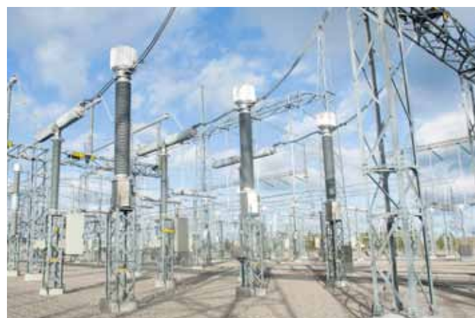
Current transformer IMB 420. Installation in Sweden.
