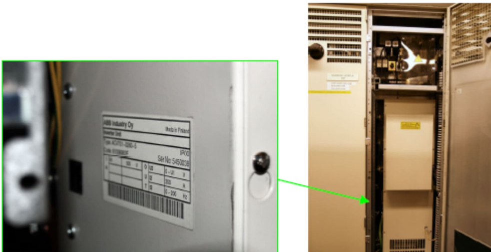
Pic 7. Inverter module of ACV700, ACV701-0250-5 (250kVA, 500V)
