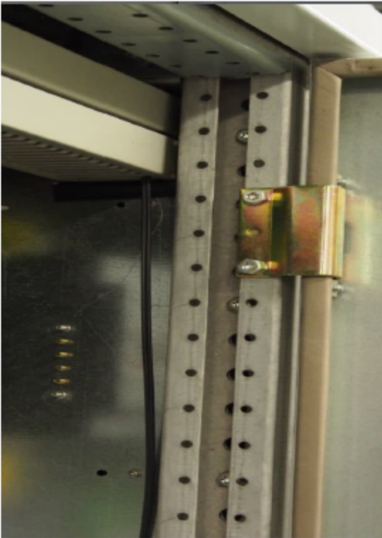
Pic 32. / 20.1. ACS600 Hole pattern of the cabinet frame
