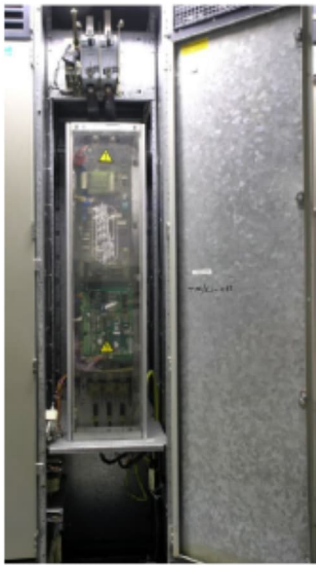
Pic 18. 400mm drive section
