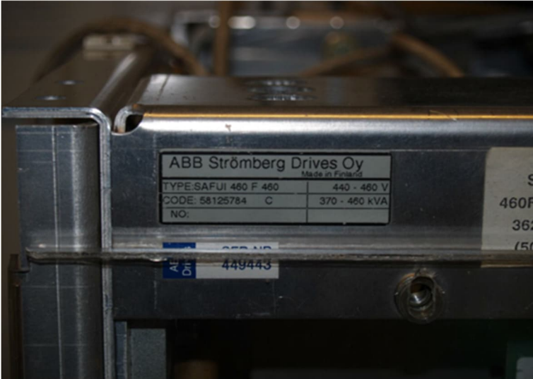
Pic 6. SAMI STAR inverter unit: SAFUI
