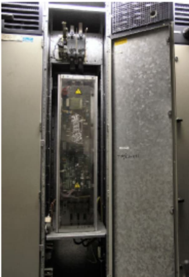
Pic 16. Older gen MD cabinet drive section
