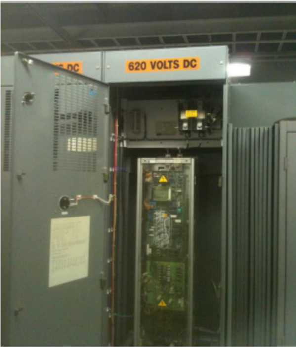
Pic 27. AB-S drive section
